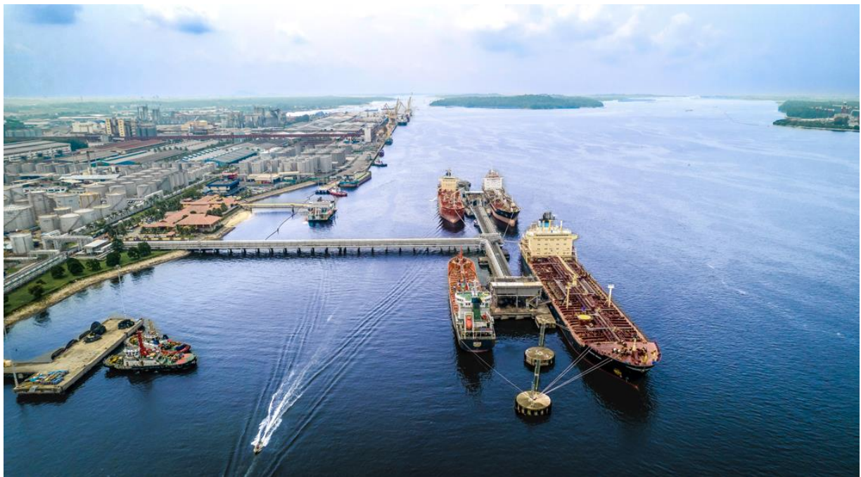
Photo caption: Aerial view of Johor Port
